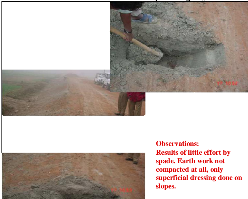
Photographs showing poor earth work in embankment
