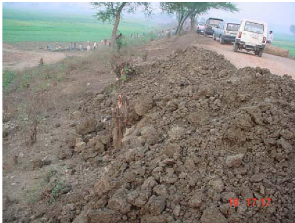
Photographs showing poor earth work in embankment
